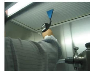
Validation service ULPA/HEPA Filter Integrity (DOP) Test
